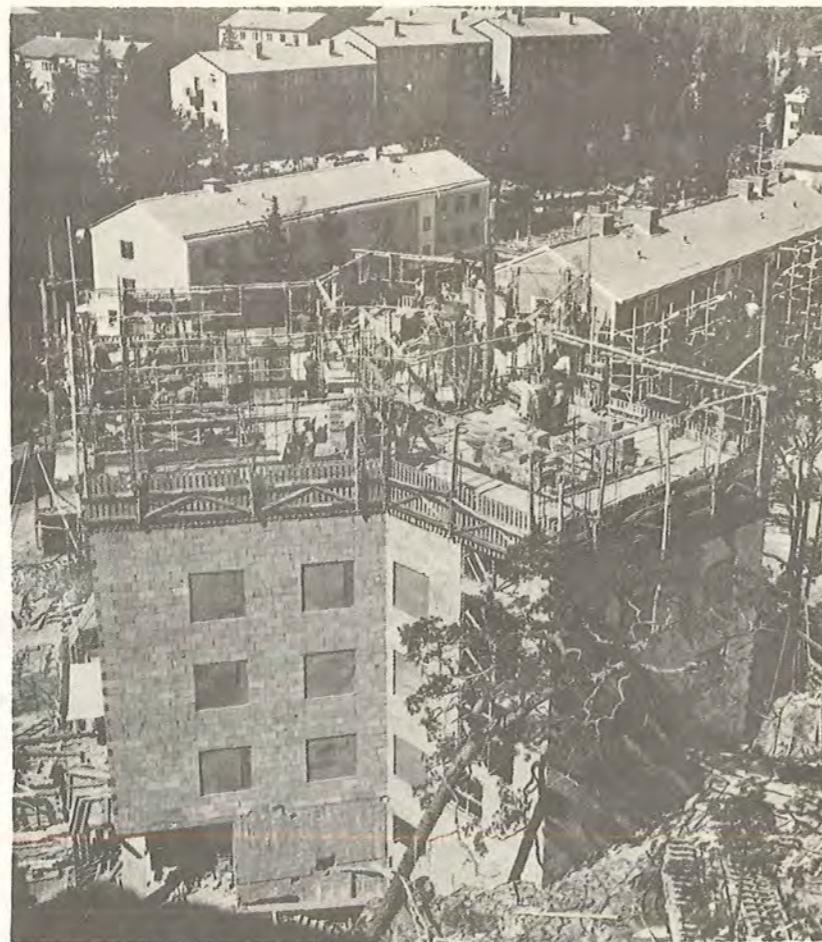
Fig. 84 Glideform. System CONCRETOR-PROMETO.
